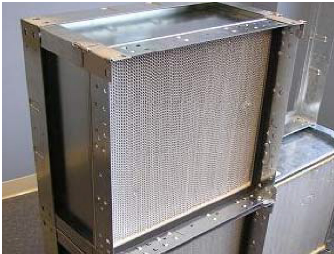
Figure 53: Properly Installed HEPA Filter
